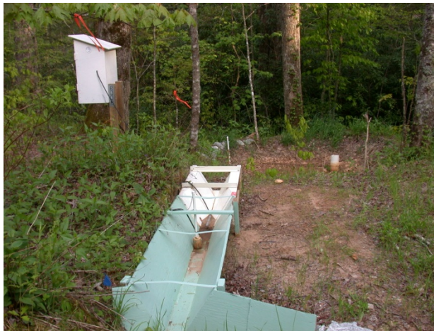
Figure 3. Inlet sampling station in road erosion and sediment control investigation. Sediment basin with riser control treatment illustrated here.
